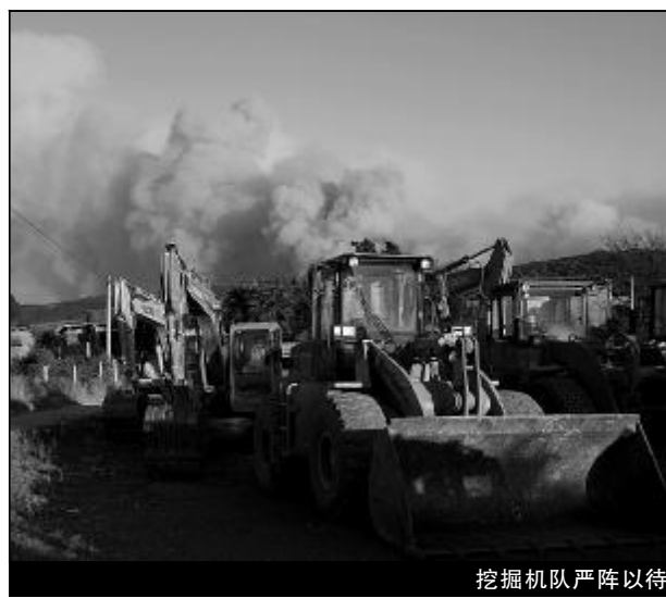
挖掘机队严阵以待
